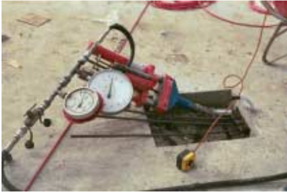
Figure 4 – Stressing pocket allows main slab pour to extend to wall.
