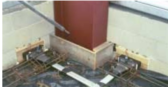
Figure 7 – Stressing access via omitted blocks in external blockwork wall
