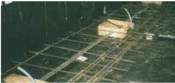
Figure 5 – Perimeter reinforcement required with stressing pockets
