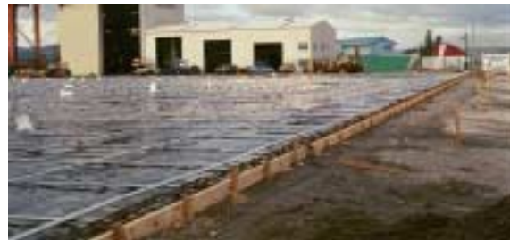
Figure 3 – Slab construction prior to erection of main structure (Port of Tauranga).
