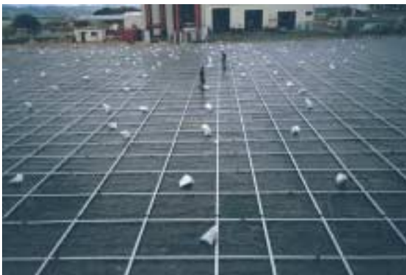
Figure 10 – Preparation of 92 m x 75 m PT slab for Port of Tauranga
