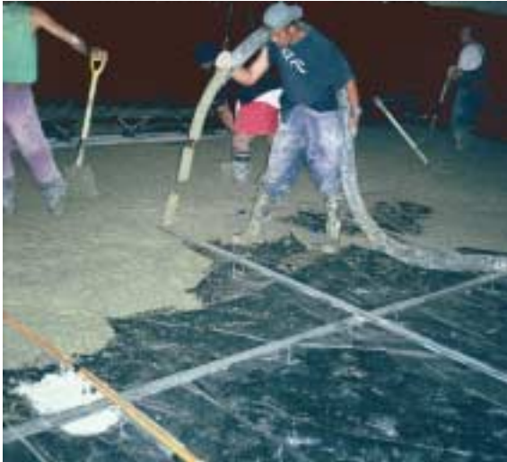
Figure 12 – Kings Wharf Coldstore
