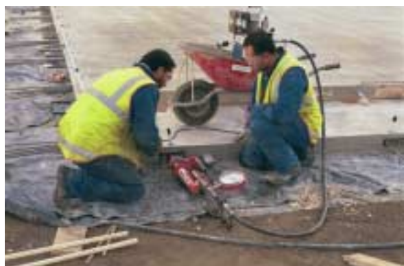
Figure 11 – Tendon stressing from slab edge
