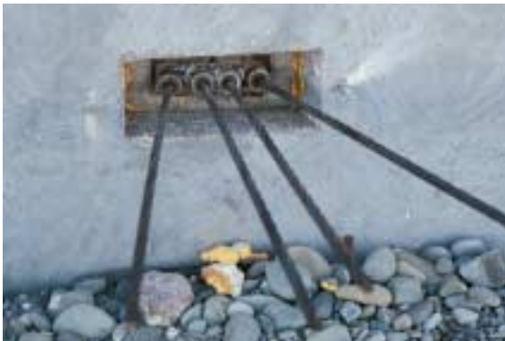
Figure 6 – Stressing access via slots in wall panel
