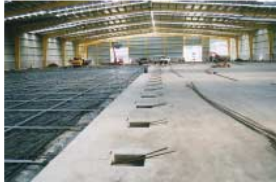
Figure 14 – Shed R at CentrePort, Wellington
